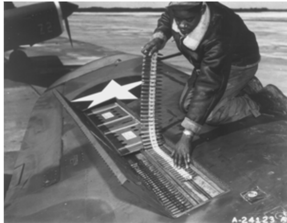
Loading .50 caliber machine gun rounds into an AAF fighter. (Courtesy National Air & Space Museum, Smithsonian Institution)
