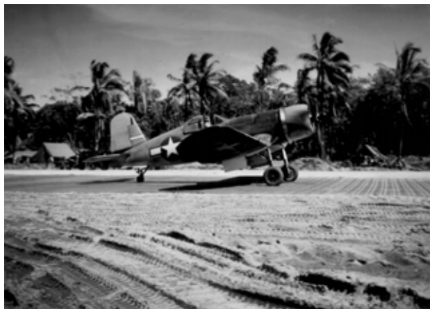
A Marine Corsair on an airstrip carved out of the jungle. By 1944, American Sea Bees and U.S. Army Combat Engineers could construct an airfield in only a few weeks. (Courtesy Bob Lawson)
