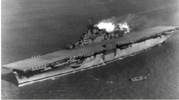
An Essex class carrier under steam. During the last phases of the war, the Essex's wooden decks proved to be highly vulnerable to kamikaze attacks. Many were seriously damaged. (Courtesy National Air & Space Museum, Smithsonian Institution)
